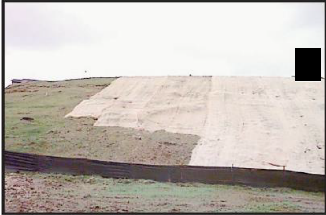
Plate 3 – Coconut matting and silt fence (Source: CIRIA, 2006 10 )
