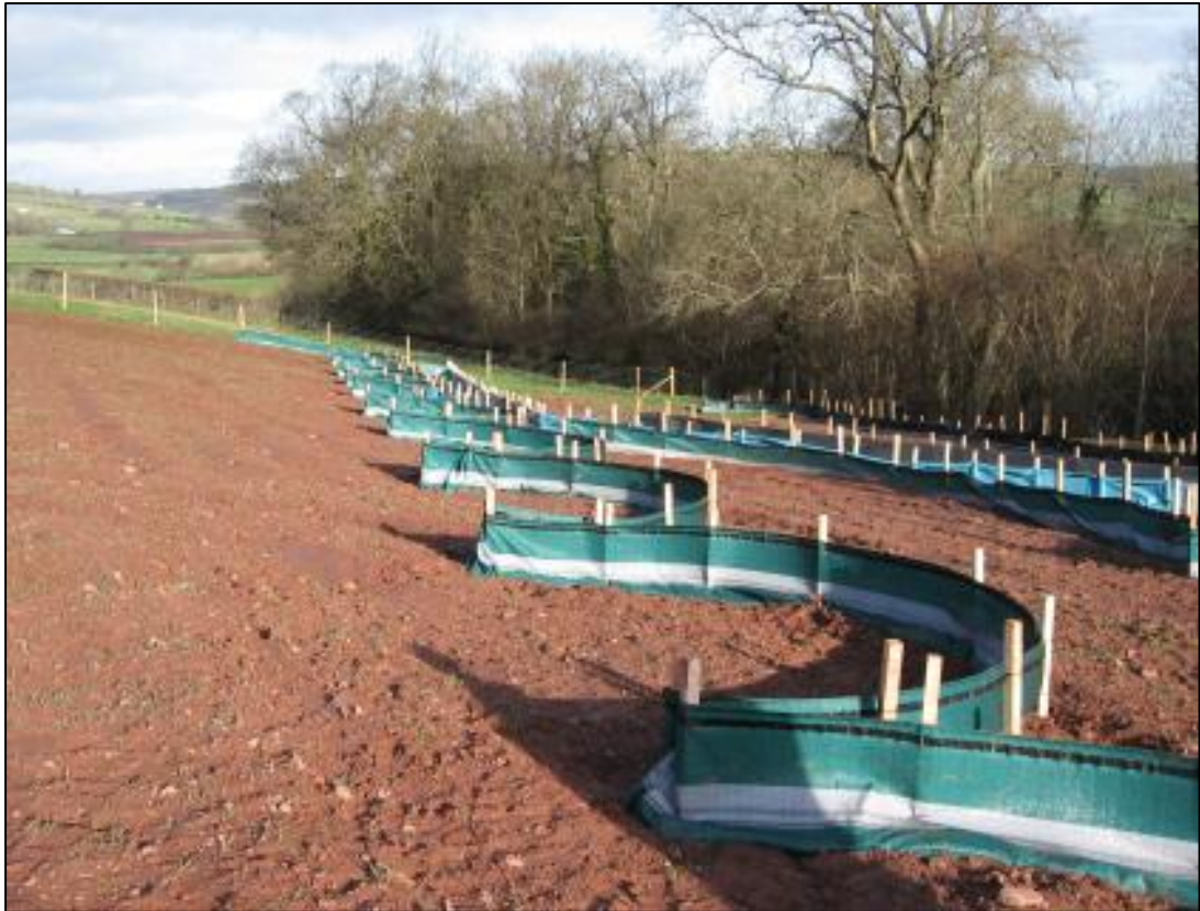
Plate 2 – Example of good practice in silt fence installation (Source: Geosynthetics, 2021 12 )
